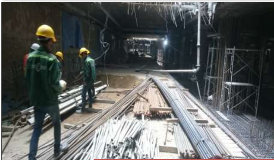
Material transfer to Basement 4 through slab opening
