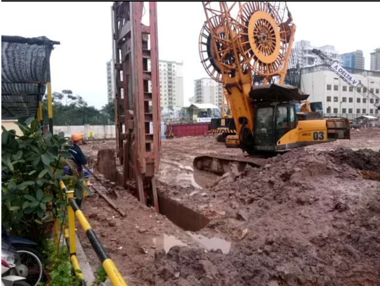
Excavation of Diaphragm Wall
