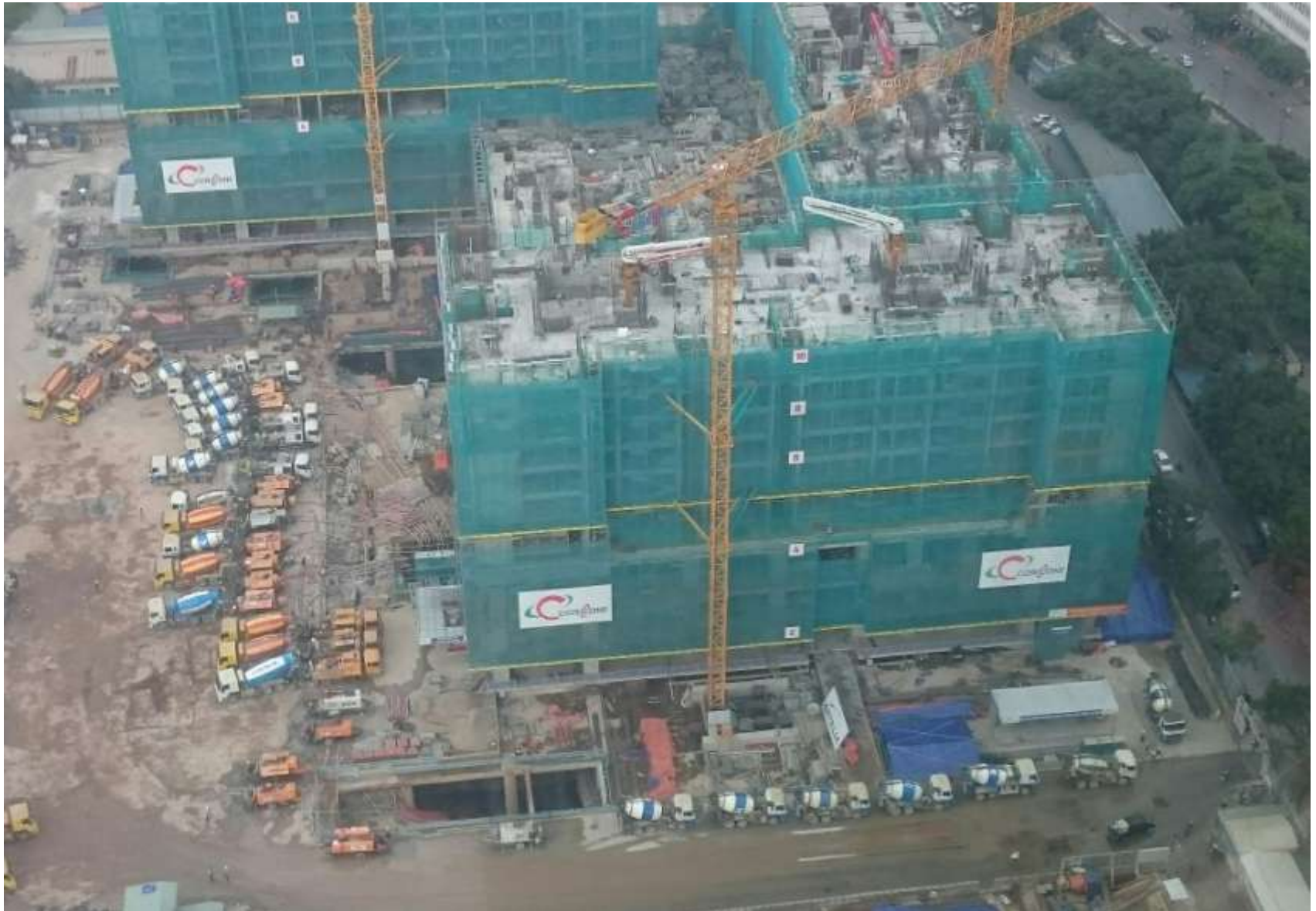
Aerial View/setting out of Concrete Mixers
