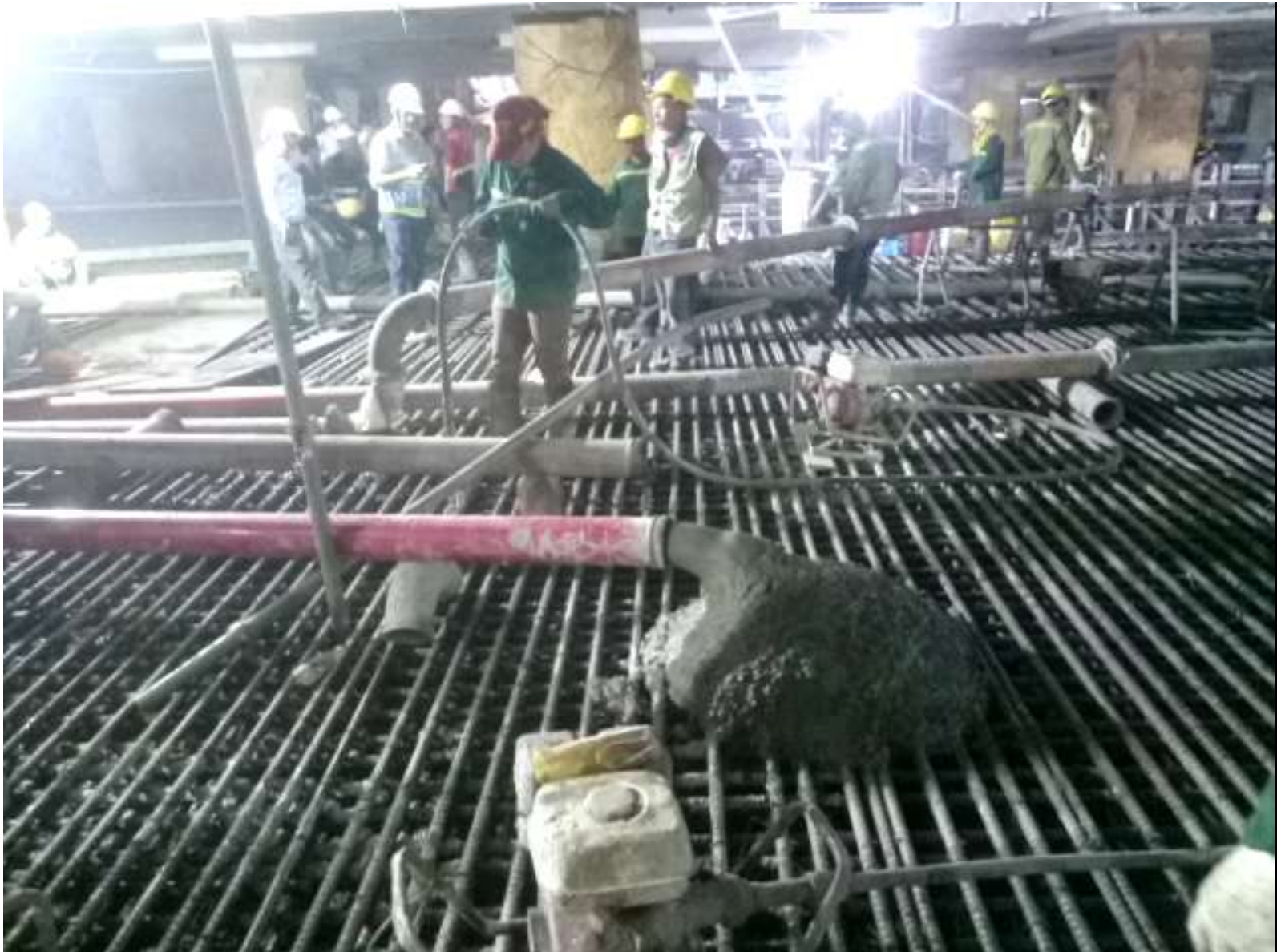
Casting Foundation Slab@top down
