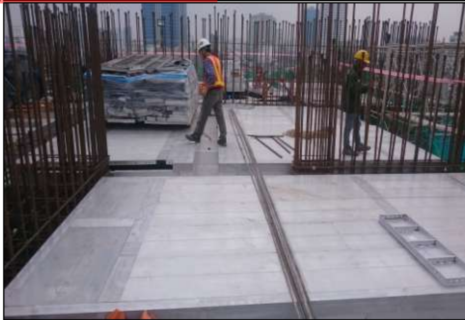
Alounimun Formwork and Scaffolding for Typical Floor L5-L45
