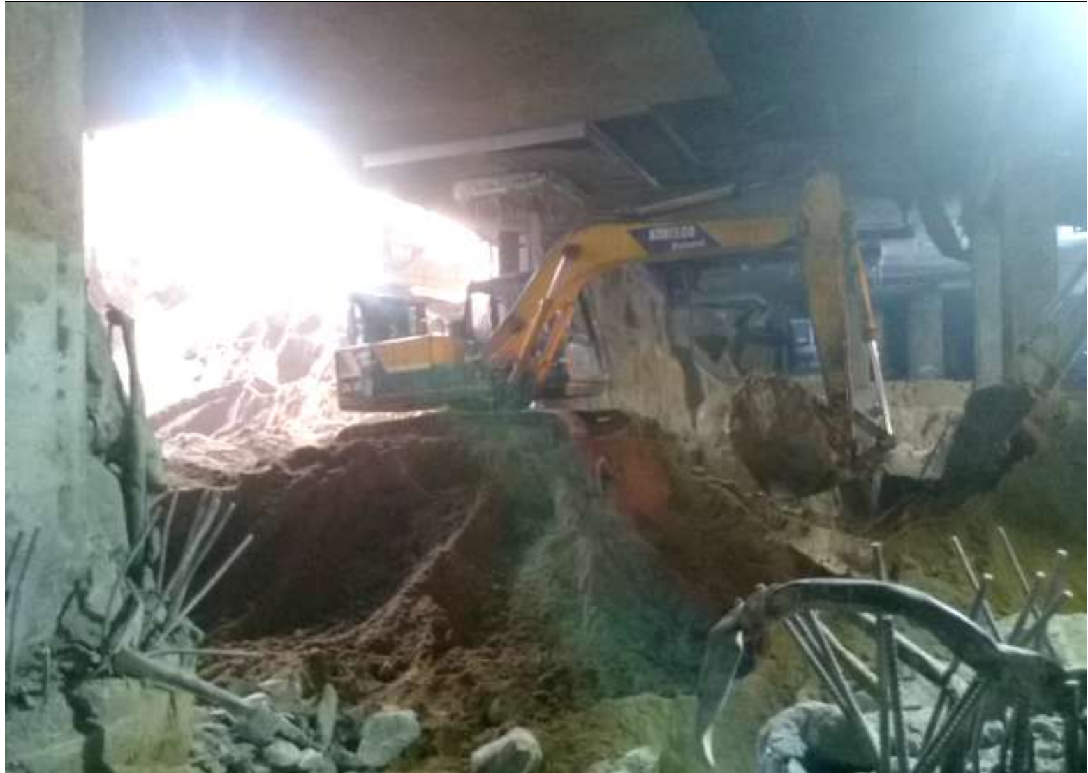
Excavation for Basement B4 and foundation slab@Top Down
