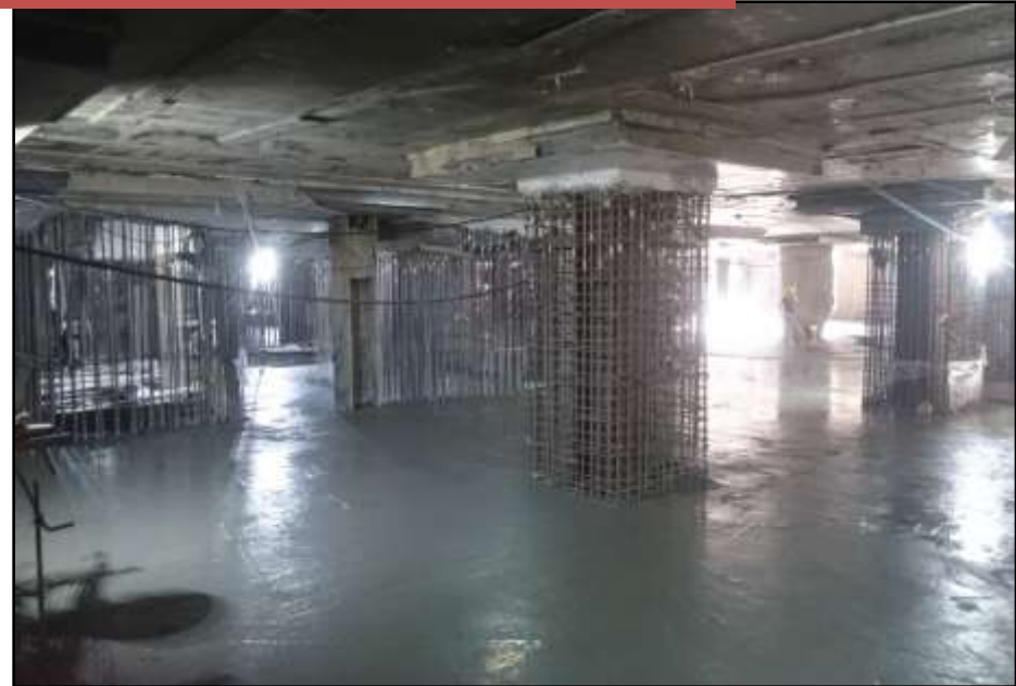
Casting Foundation Slab Mass Concrete
