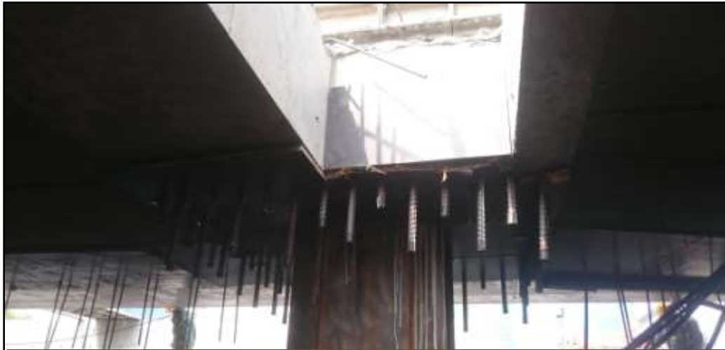
Starter bars for connection with RC Column Bars
