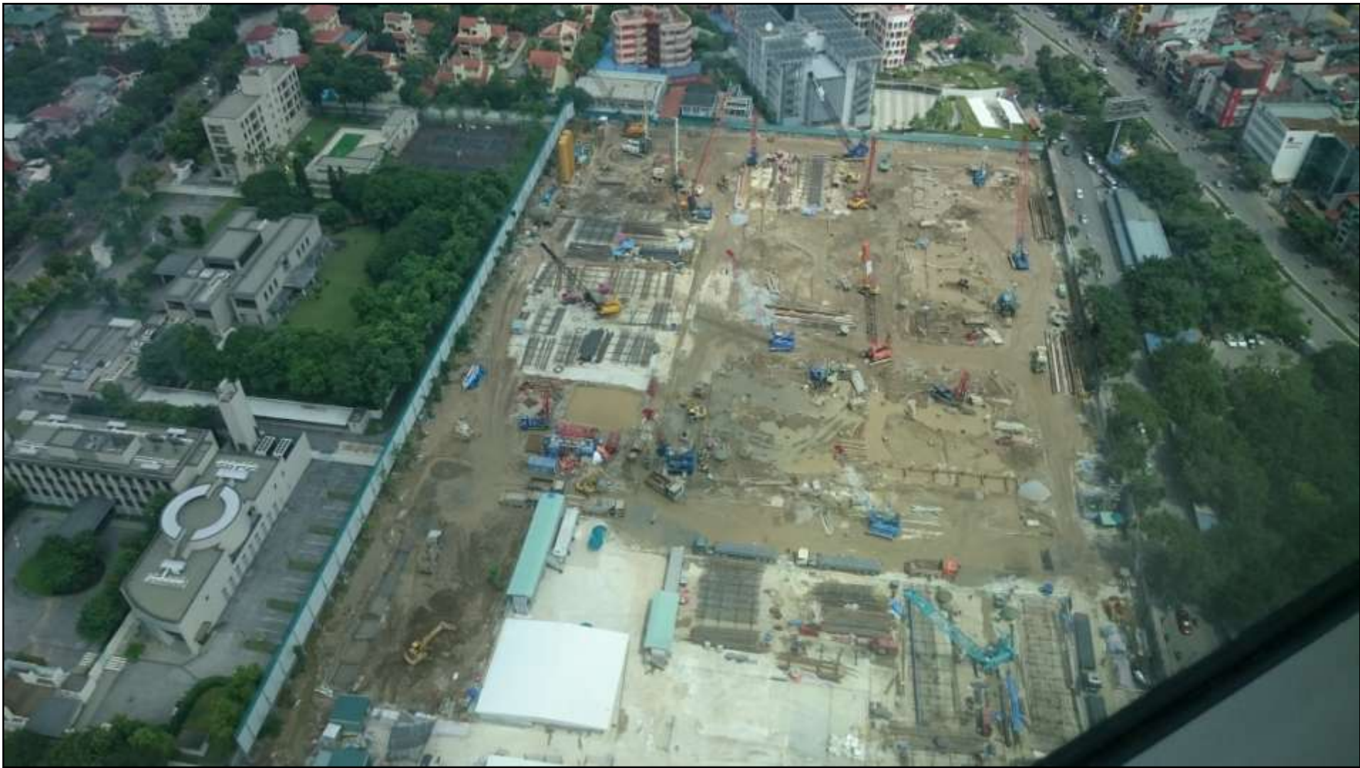
Aerial View from Site – Piling Equipment Mobilization
