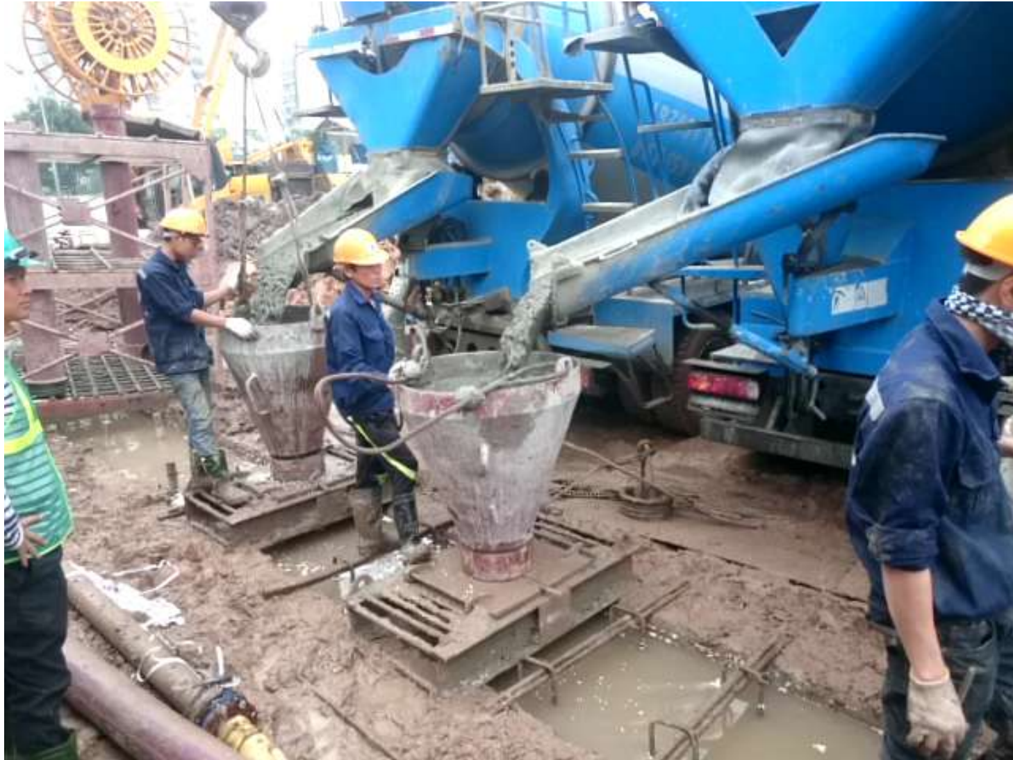
Casting of Diaphragm Wall
