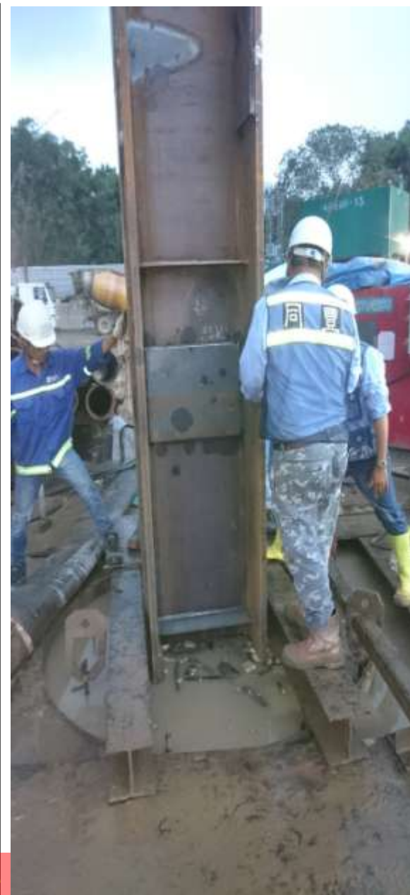
King post installation on top of pile
