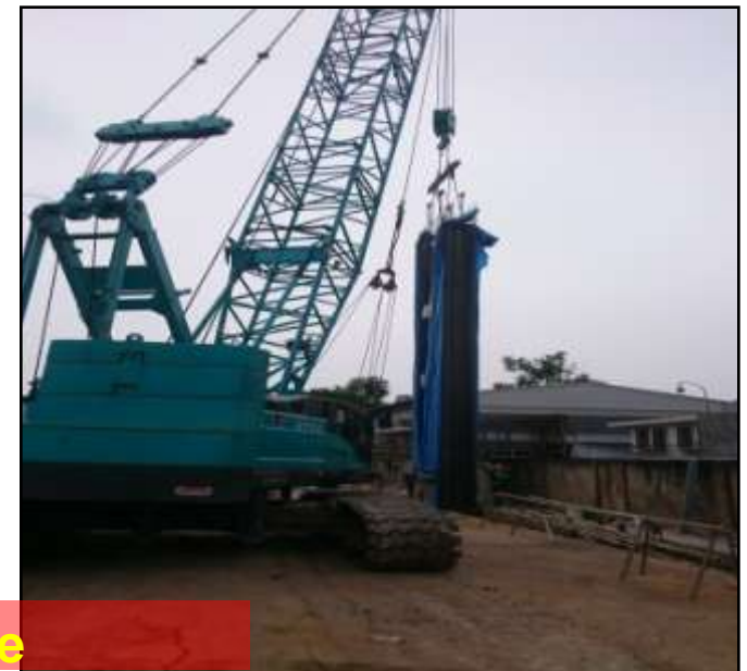
Excavation for Diaphragm Wall of Basement
