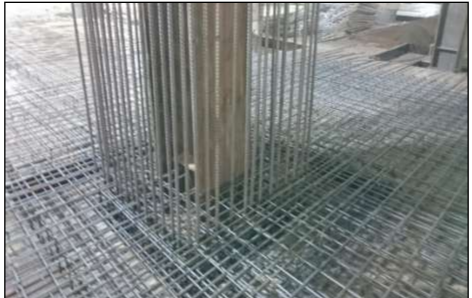
Installation of reinforcement of slab
