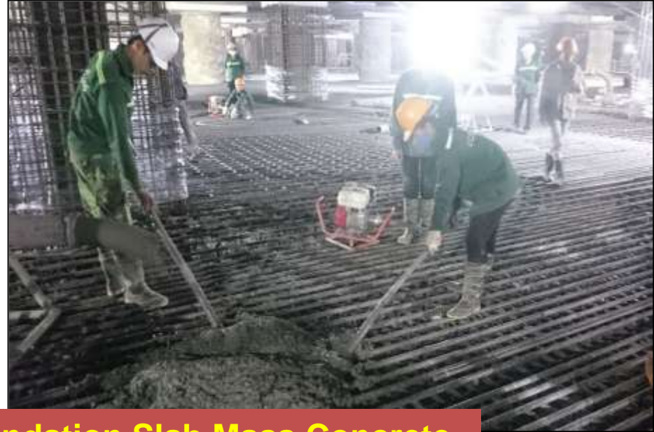
Casting Foundation Slab Mass Concrete
