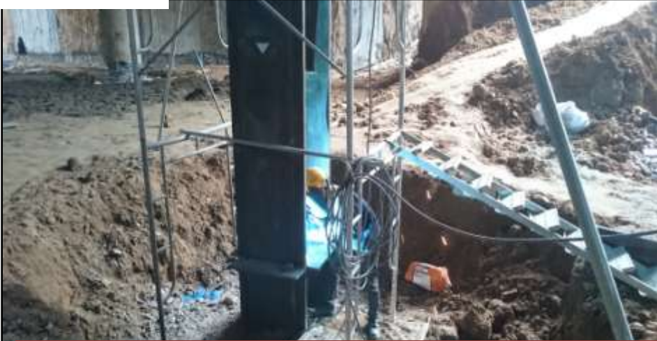
Welding Steel Plates for King Post Connection to RC Beam
