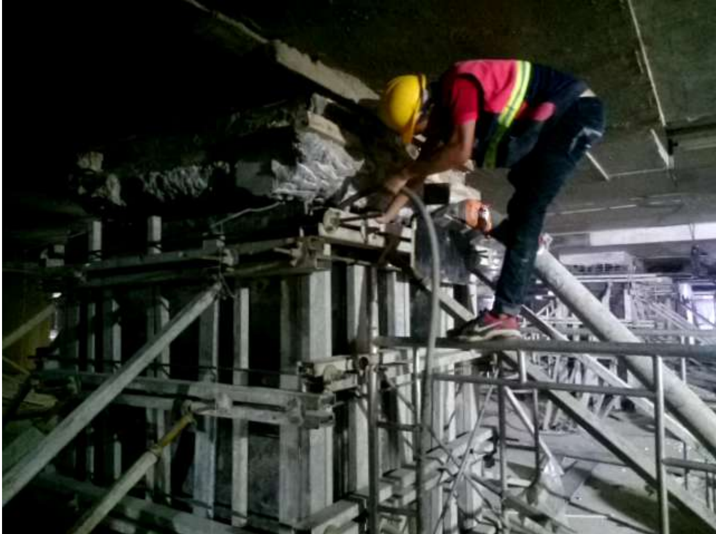
Casting RC Columns/Walls, encasing the King Post
