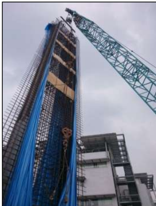
Pile Reinforcement Cages
