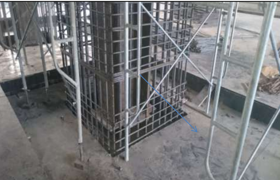
Installation of rebar for columns top down
