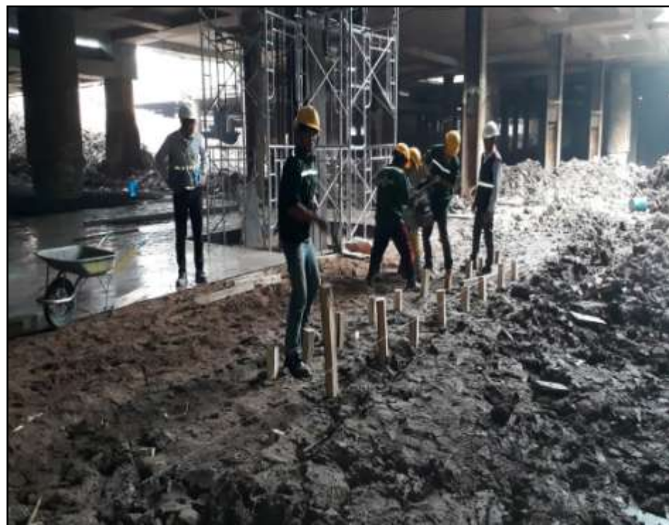
Installation of Wood Post for Soil Improvement
