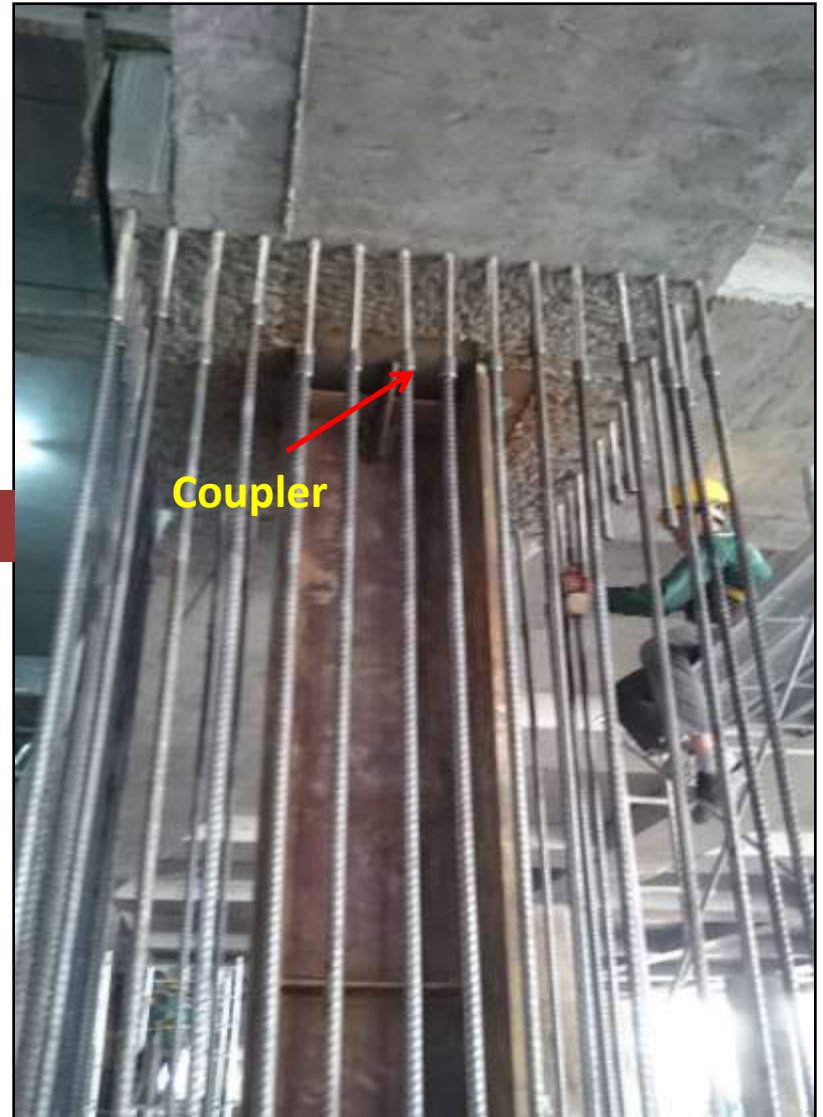
Fixing reinforcement from top to bottom
