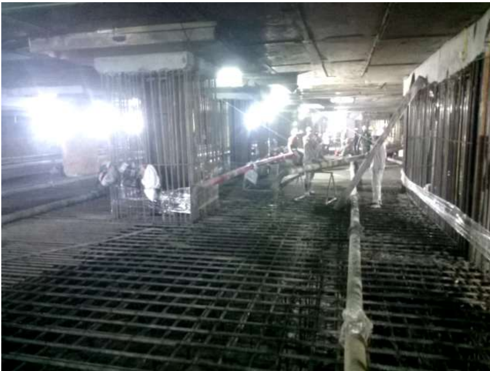
Casting Foundation Slab@top down
