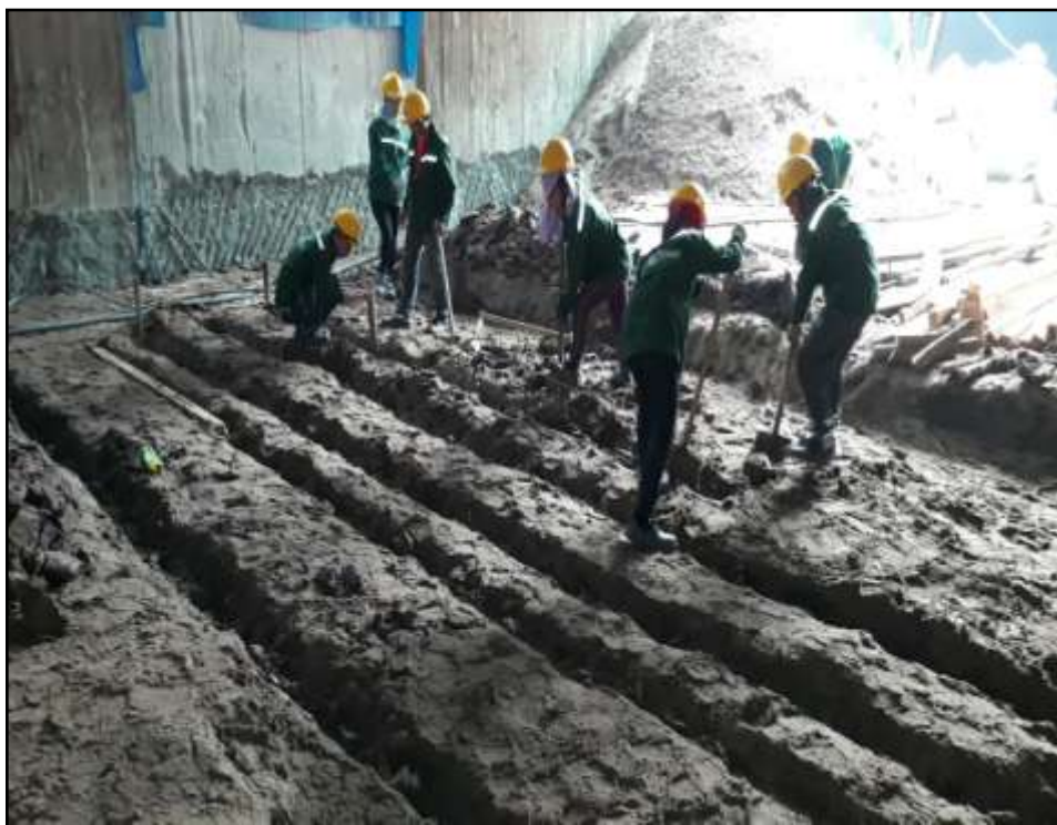
Installation of Wood Post for Soil Improvement
