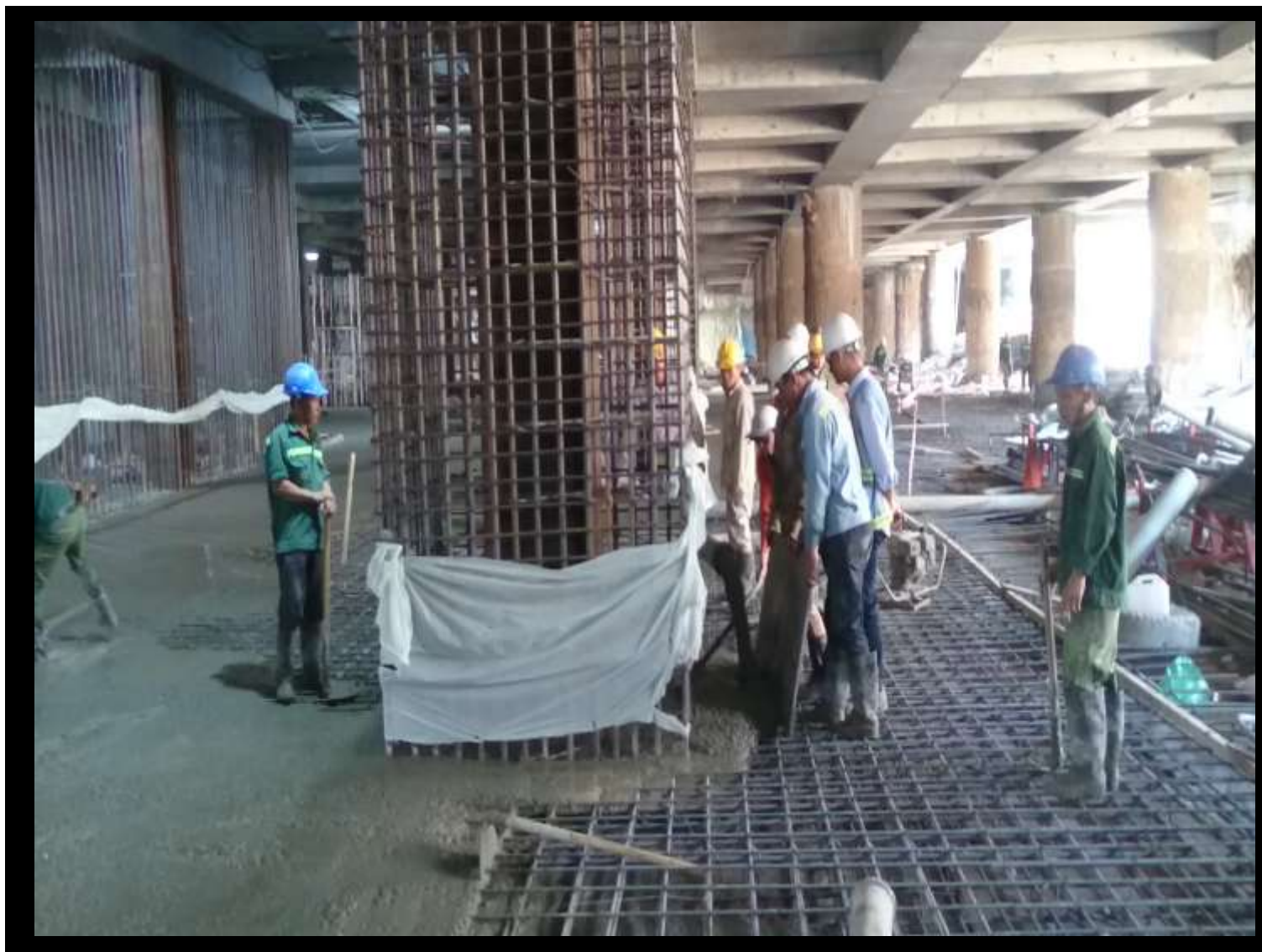
Casting Basement B1 Slab@Top Down
