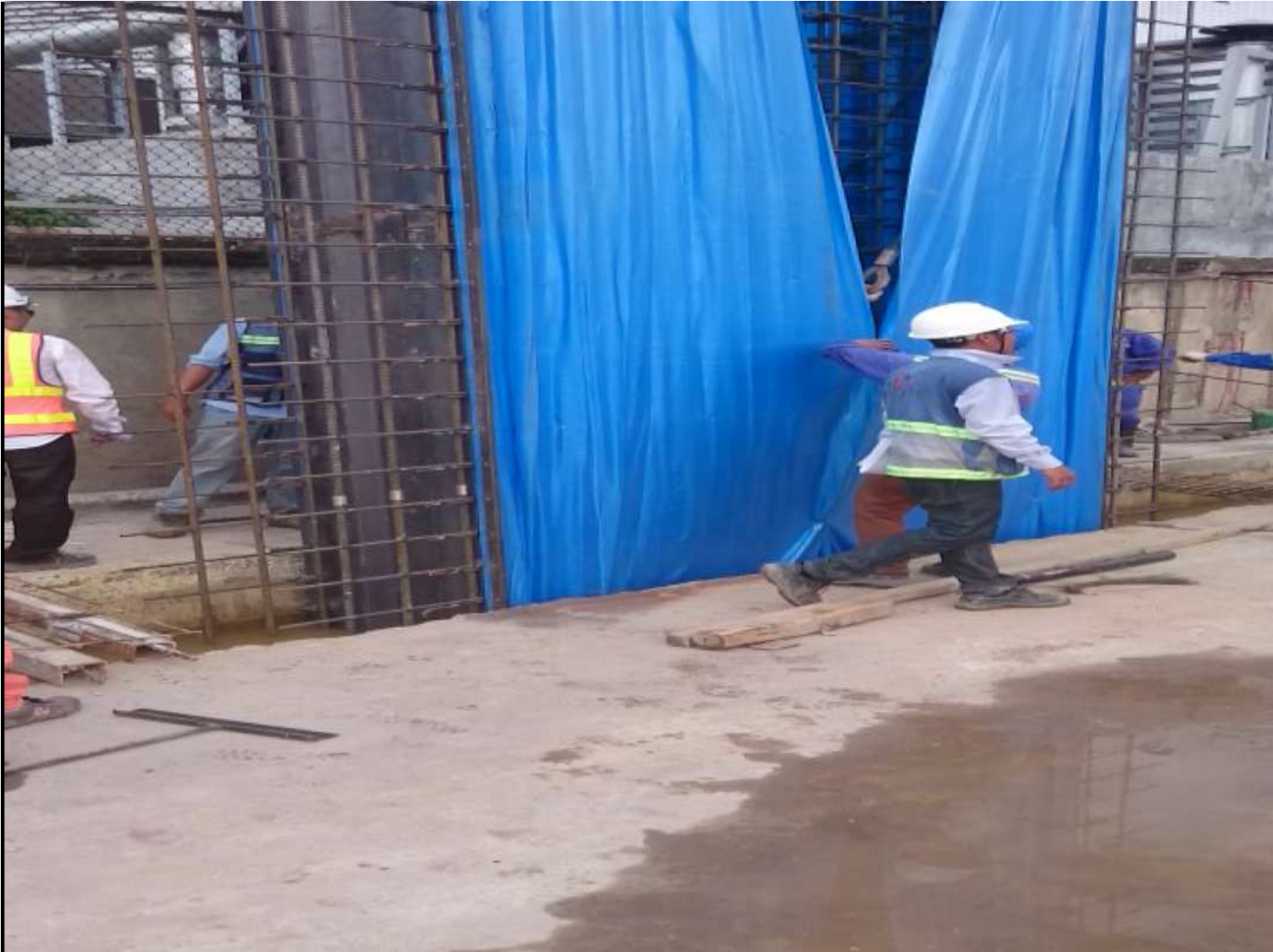
Installation of Reinforcement Cage - Diaphragm Wall
