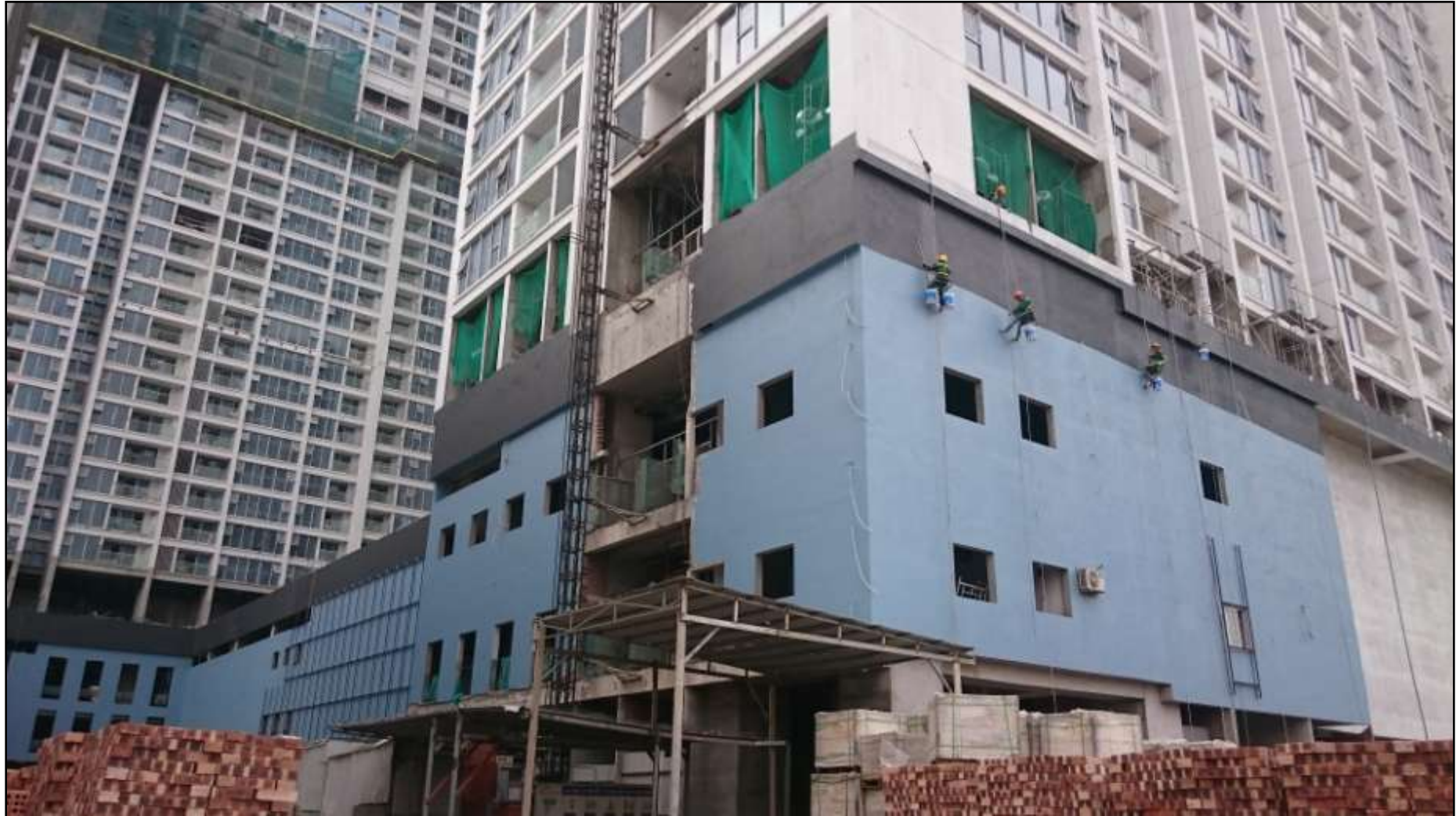
Facade at Podium – Water Barrier/ April 2018
