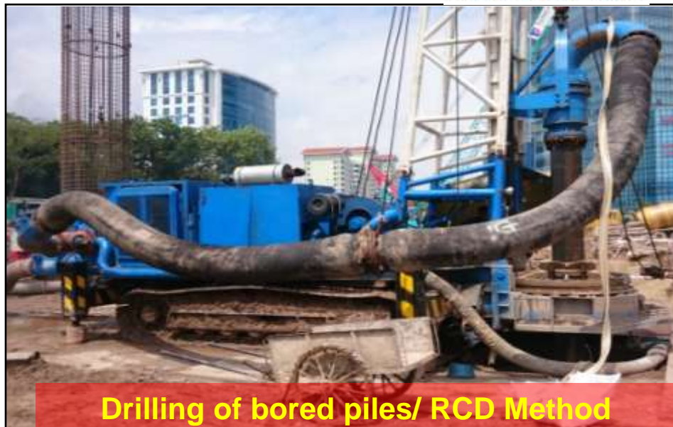
Mobilization of Equipment for piling works
