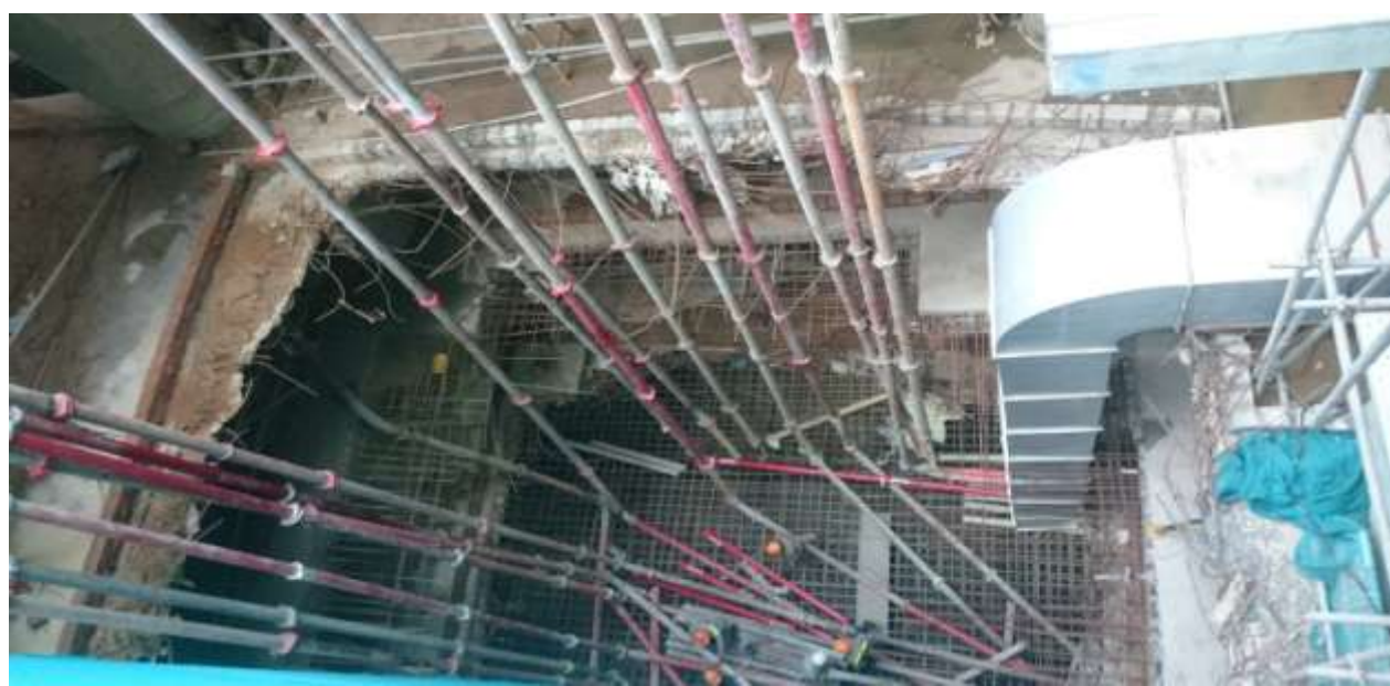
Preparation Works for Casting – Installation of Pipe Lines
