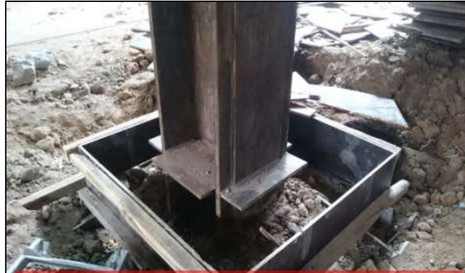
King post/RC Beam connection
