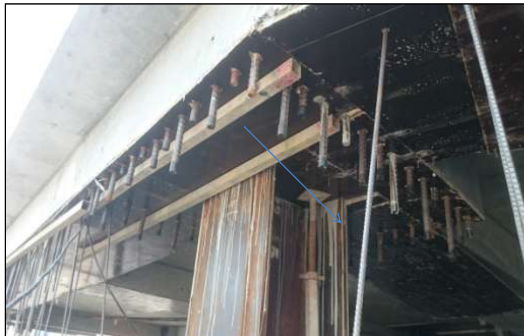
Starter bars for connection with RC Column Bars
