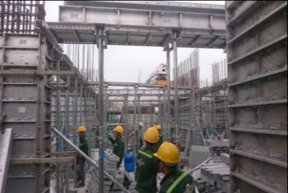
Alounimun Formwork and Scaffolding for Typical Floor L5-L45
