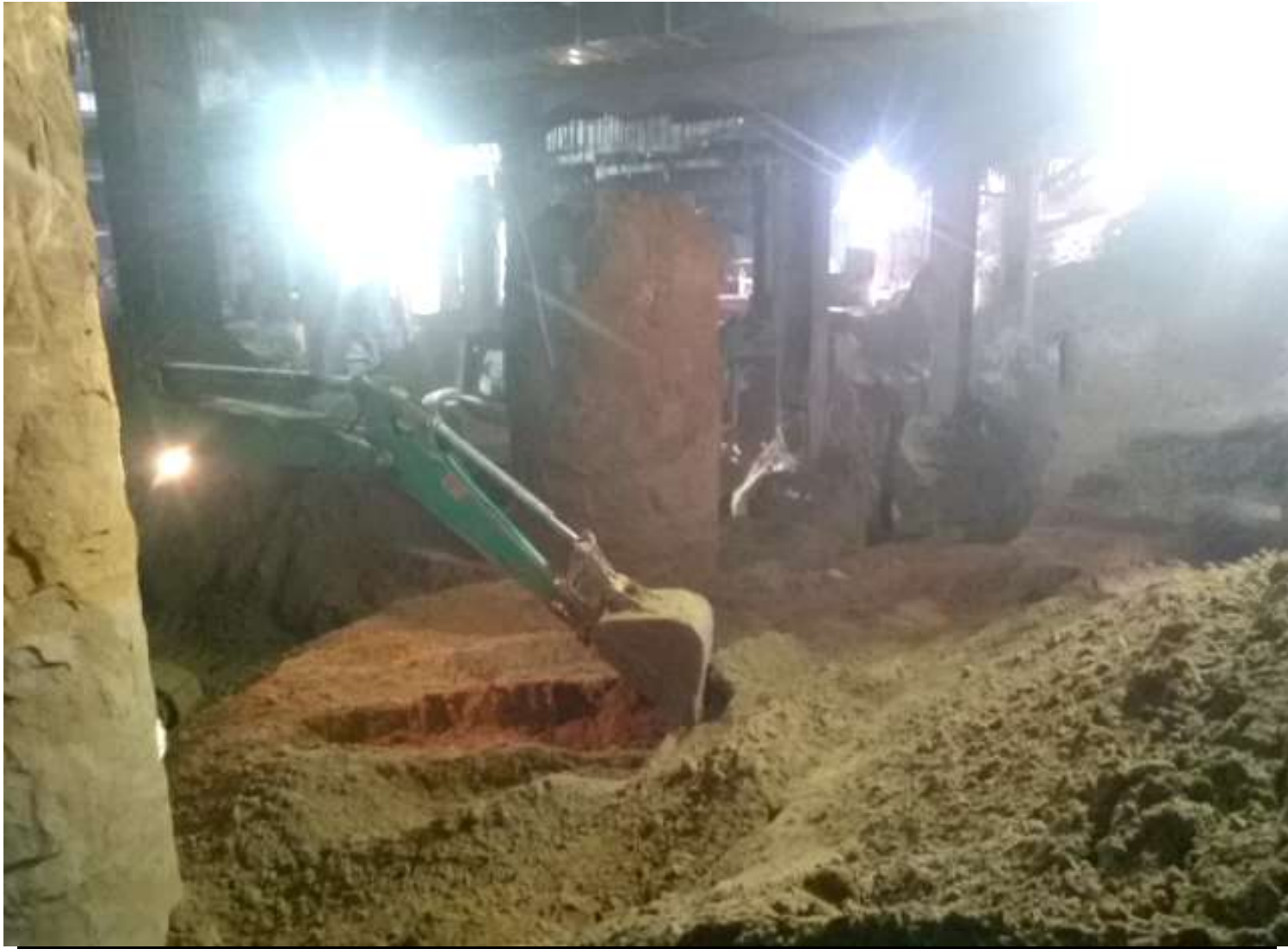
Excavation for Basement B4 and foundation slab@Top Down
