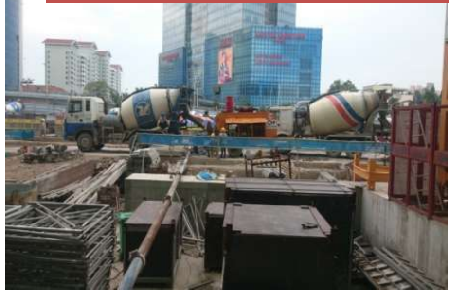
Arrival of Concrete Mixers and Start Casting Foundation Slab
