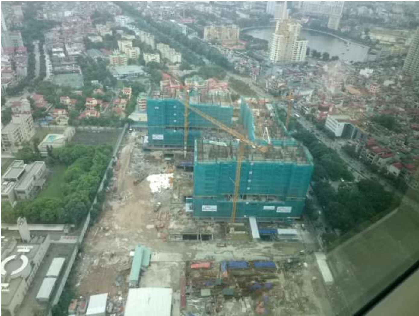
Superstructure at Level 10/ Construction of Basement B4 and Foundation
