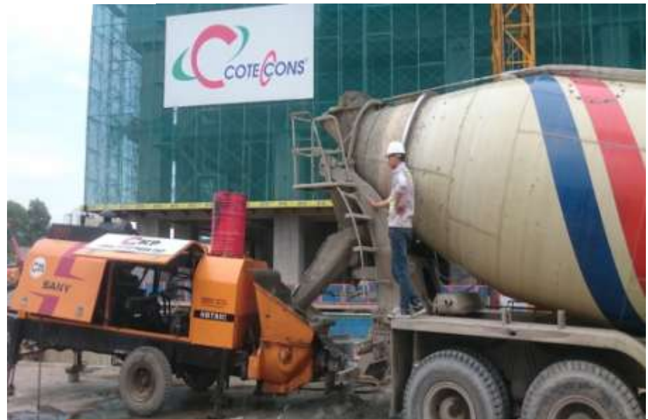
Arrival of Concrete Mixers and Start Casting Foundation Slab
