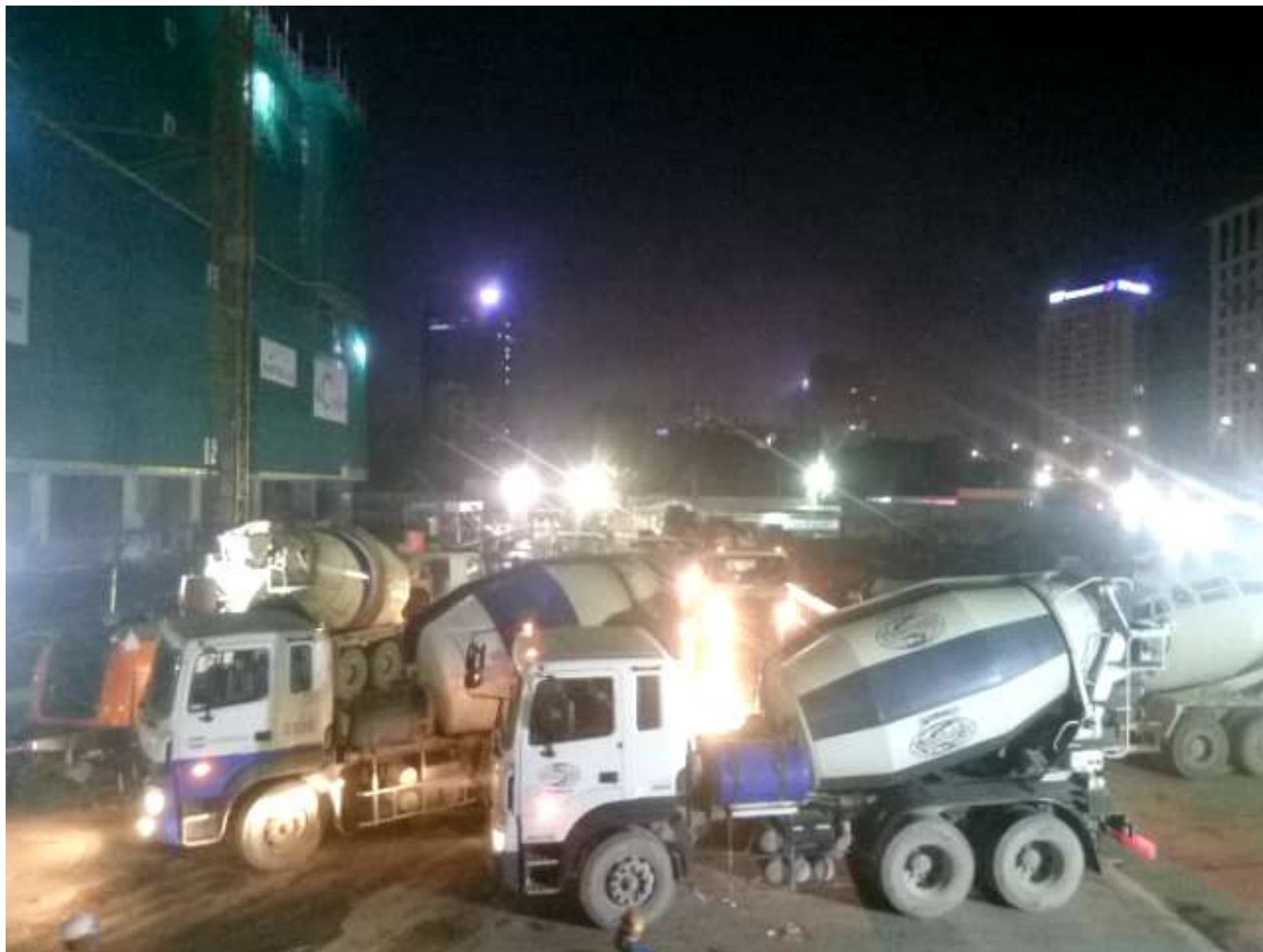
Transit Mixers arrival to site
