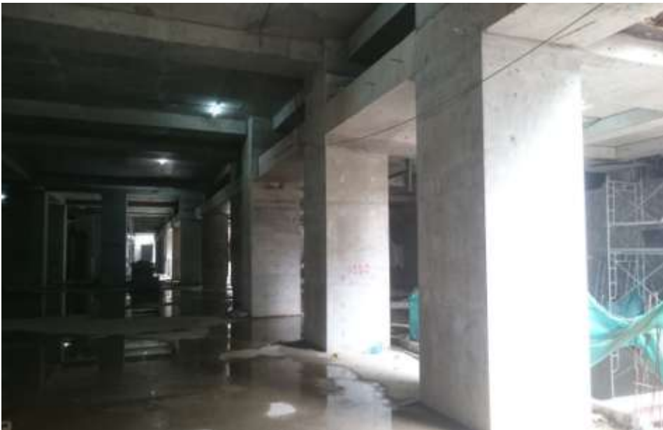
Completion of grouting for Columns/Wall
