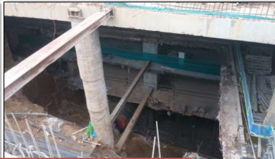
Material transfer to Basement 4 through slab opening
