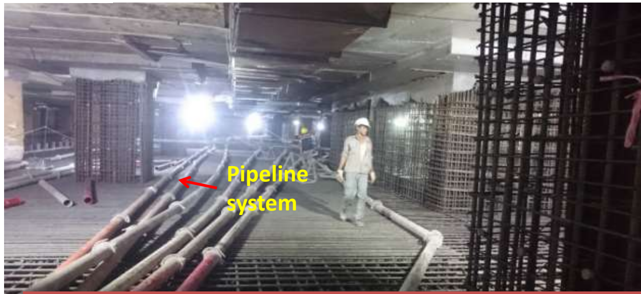
Preparation Works for Casting – Installation of Pipe Lines
