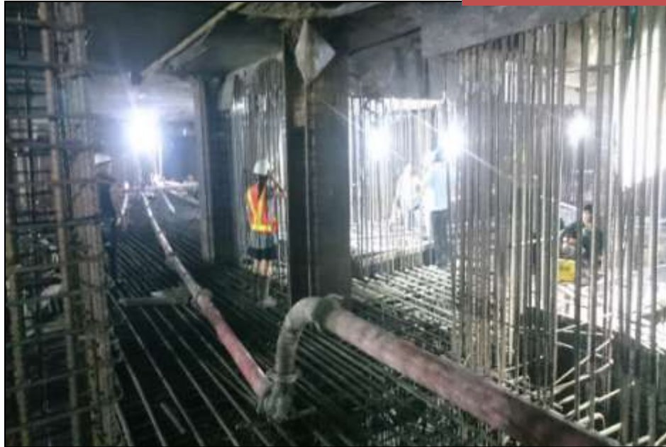
Casting Foundation Slab Mass Concrete
