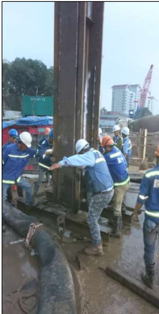
King post installation on top of pile
