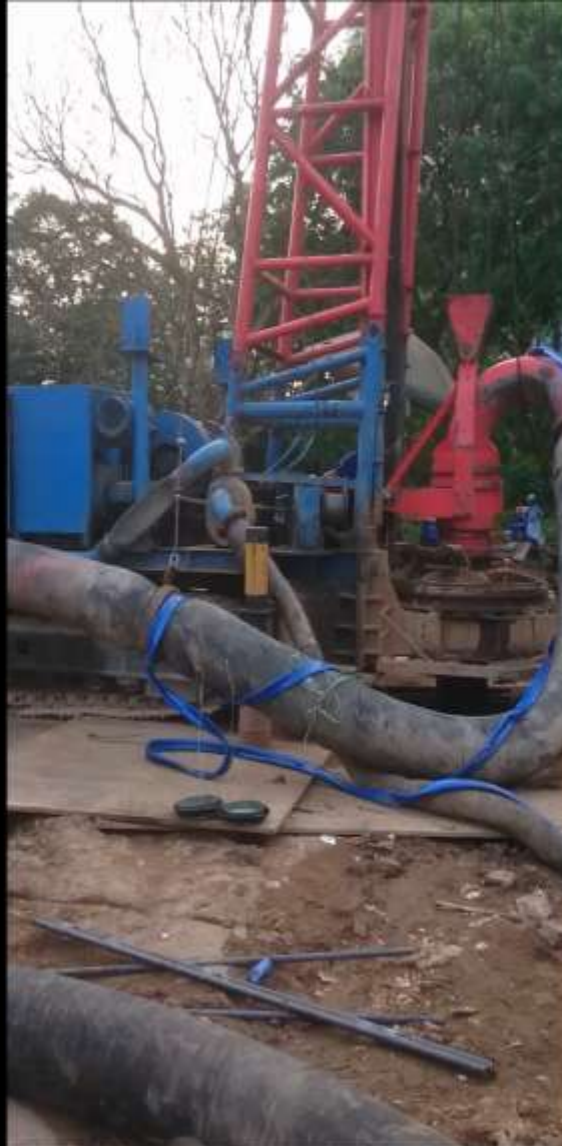
Drilling with RCD for piling
