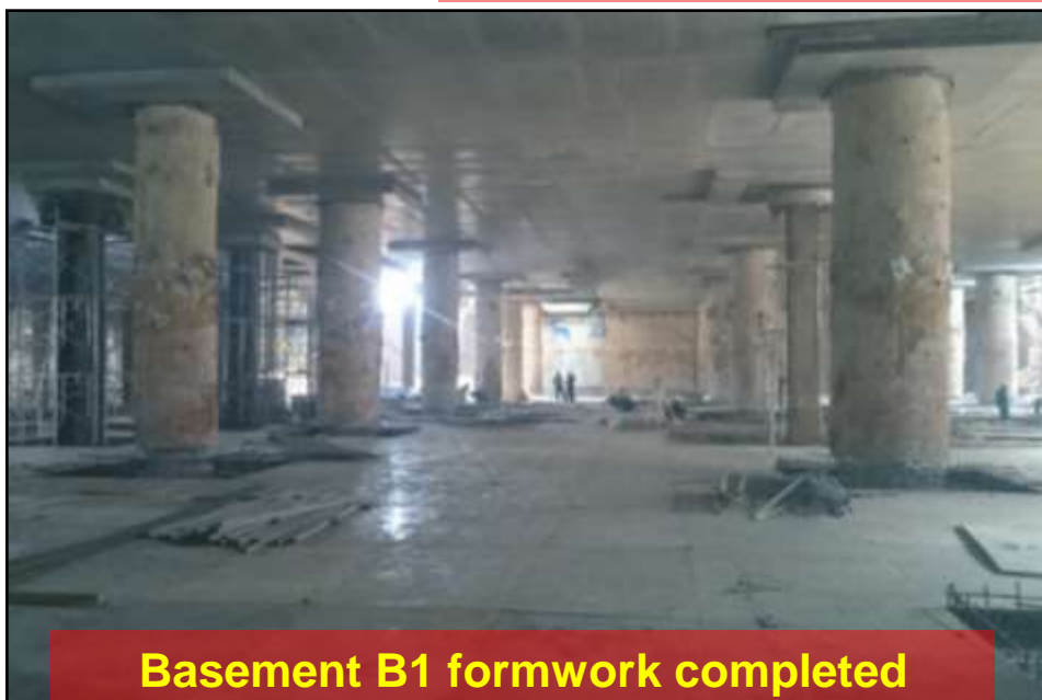
Levelling of soil and installation of formwork
