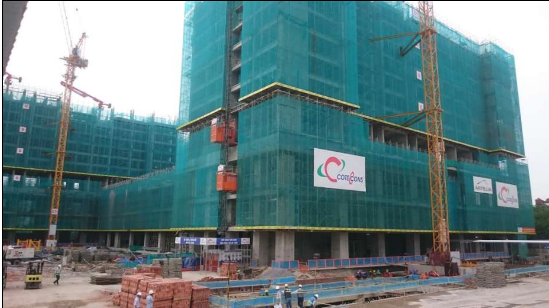
Superstructure at Level 12/ Basement B4, Foundation and RC Columns Completed
