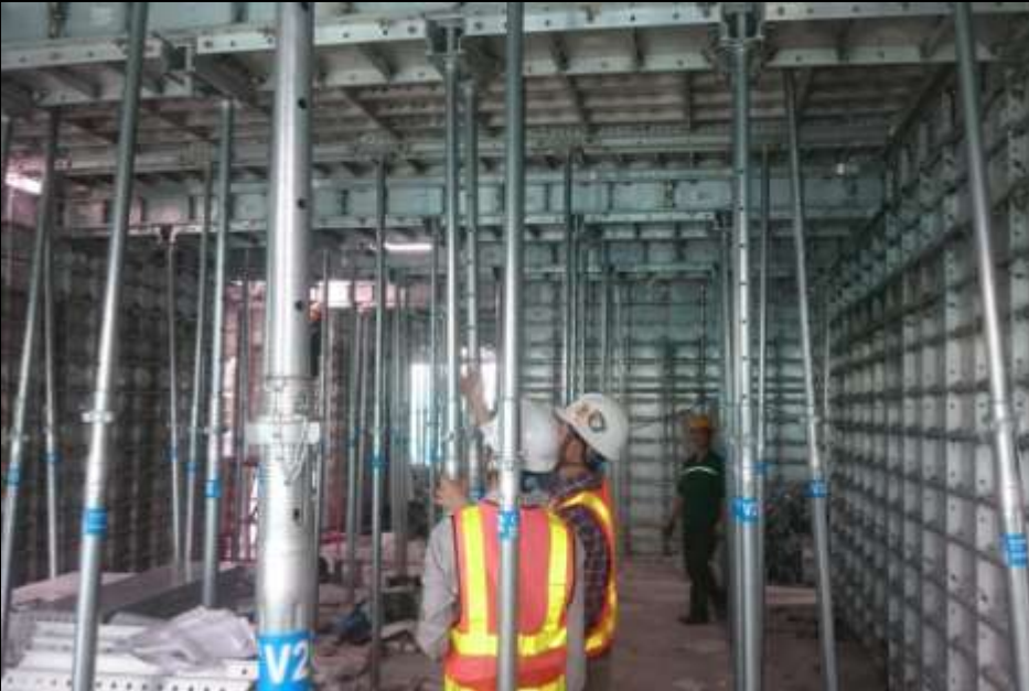
Alounimun Formwork and Scaffolding for Typical Floor L5-L45
