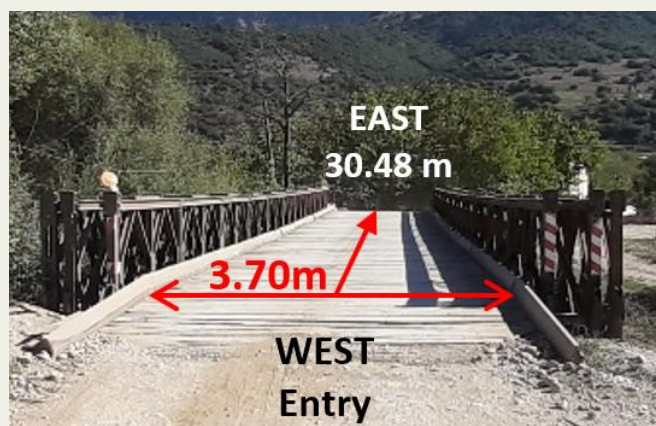
Fig. 1 The Bailey Bridge at Feneos Village
