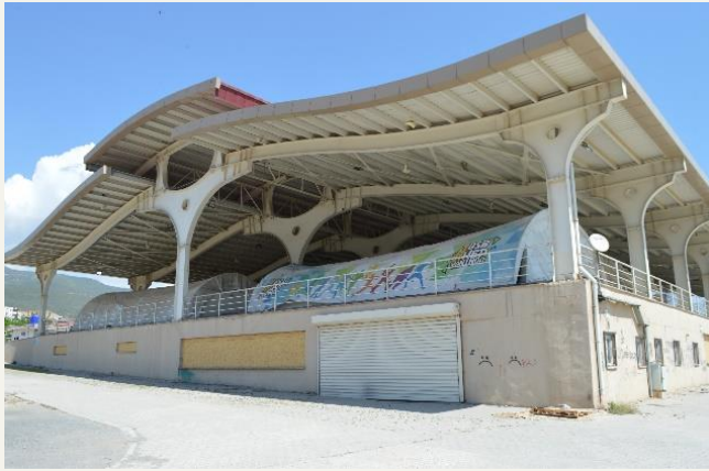
Fig. 4 Roof structure of the municipal market, Nurdaği
