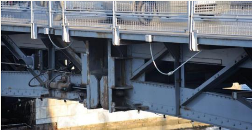
Fig. 3 Pin at the middle of the span (D1)
