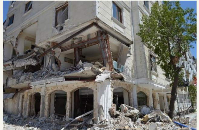
Fig. 6 Retrofitted RC building with steel members, Antakya
