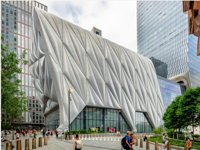
Fig. 2 The Shed in New York City, USA - The Shed is a unique cultural center that features a movable outer shell, known as the "shed," which can expand or retract to create different performance spaces. The telescoping structure allows for the creation of indoor and outdoor venues of varying sizes, accommodating a wide range of artistic and cultural events.
