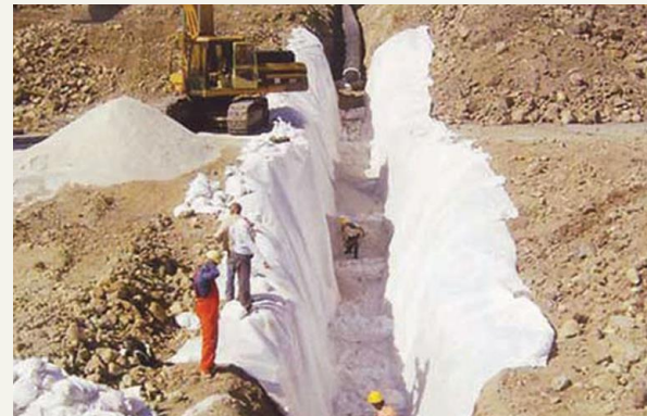
(a) Geotextile-lined trench
