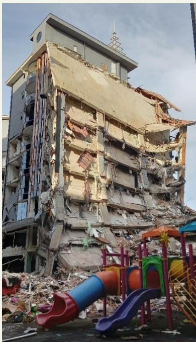
Fig. 2 Partial collapse of a 9-storey flat slab RC building, Adiyaman
