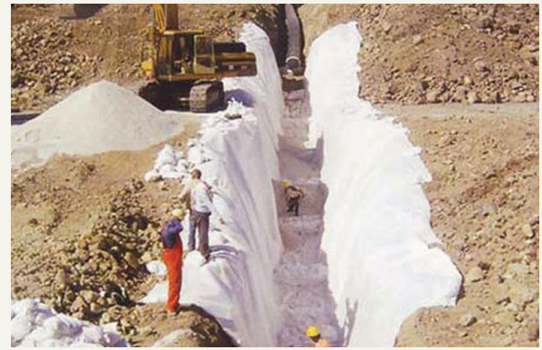
(a) Geotextile-lined trench
