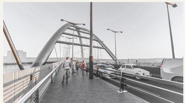
Fig. 5a Through bridge with two consecutive diagonal main arches [2x100 m] (Vasileios-Minoas Bampatsikos, MSc, 2023)
